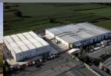
TMF - CASTELLO BRIANZA (LECCO): HYDRAULIC FITTINGS AND COMPONENTS
